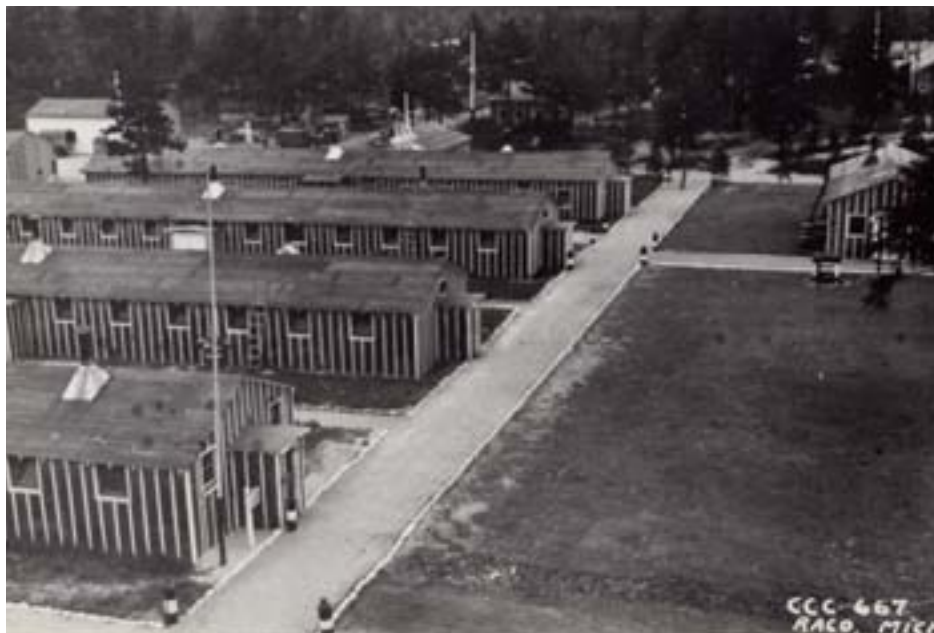
Camp Raco, was the first Civilian Conservation Corps camp created in the Upper Peninsula. Later, after the CCC was discontinued, Camp 667 was one of five in the Upper Peninsula converted to house German prisoners of war. The buildings and other structures at all of the camps looked similar, the tarpaper and lathe covering for the buildings is characteristic of the camps. (Photograph courtesy of Bernard Arbic)
